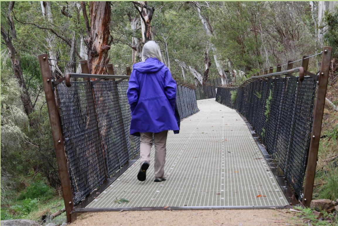
Raised platform avoiding the old rough track below (flood prone)
