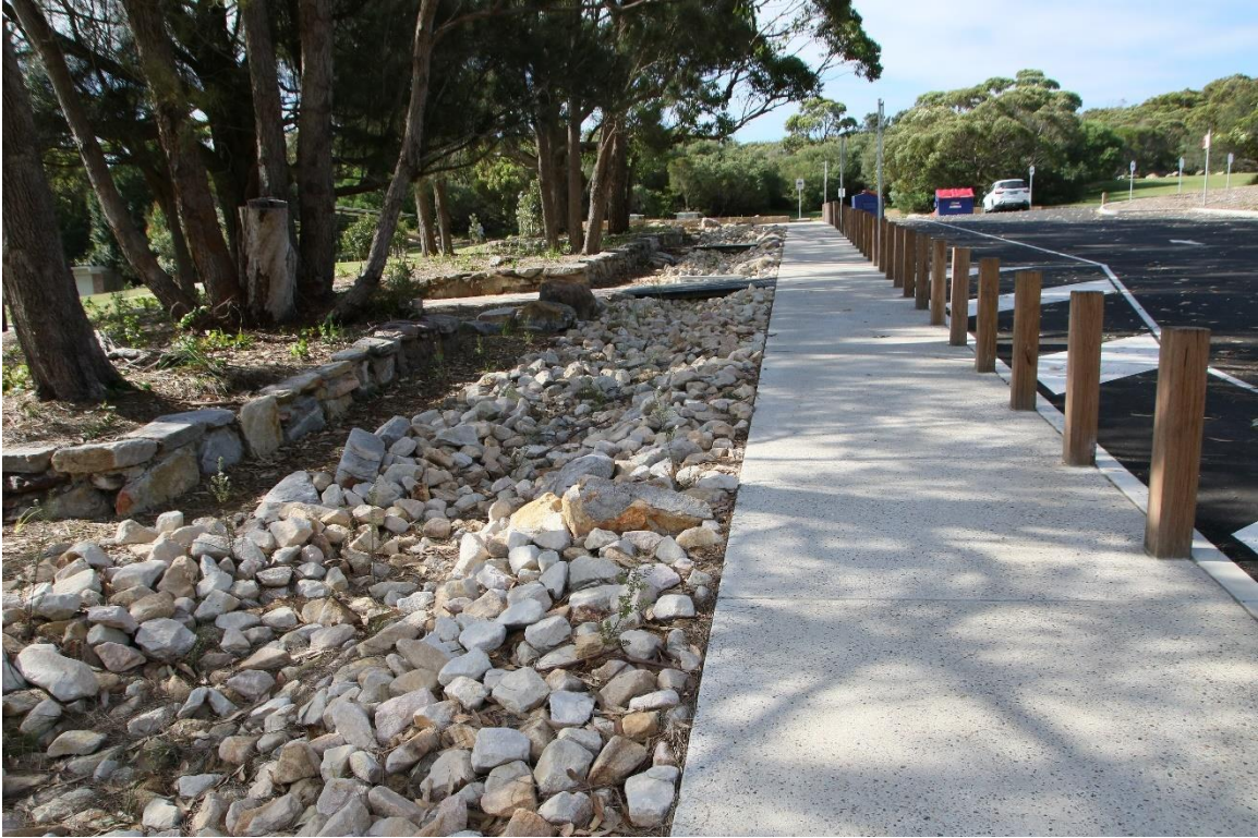
Filtered drainage lines to control and clear any water running into the creek and lagoon
