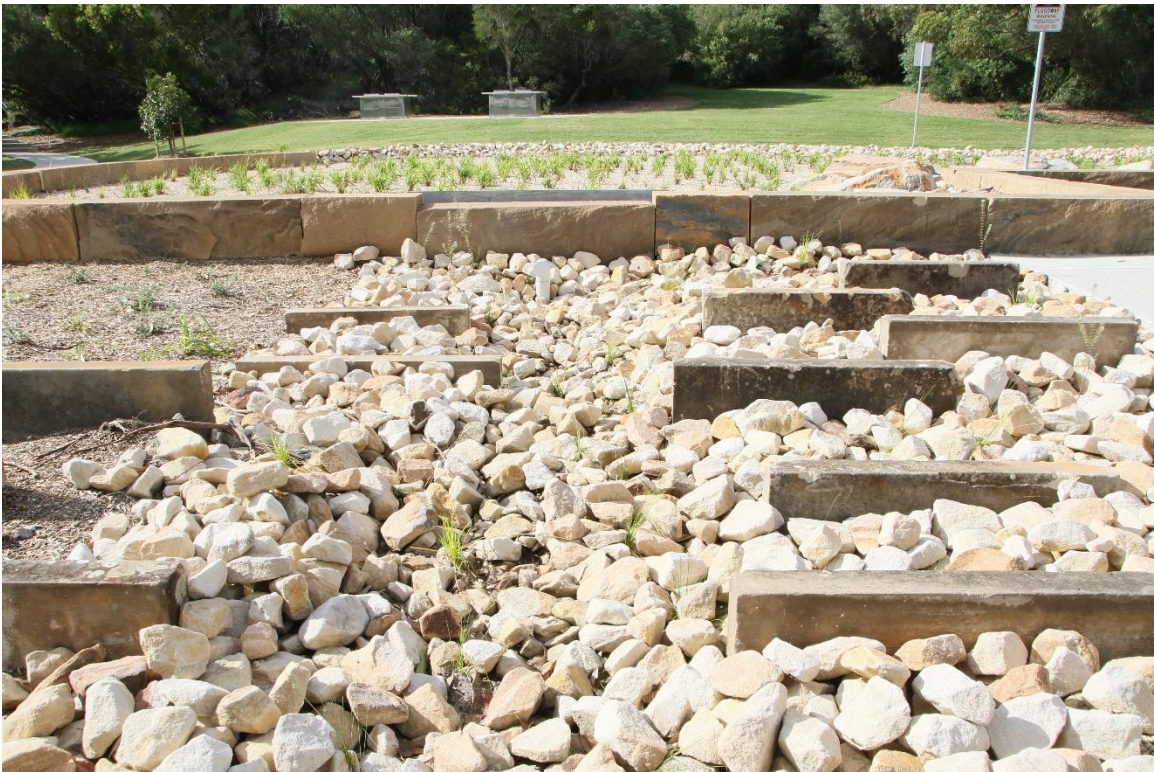
Filtered drainage lines to control and clear any water running into the creek and lagoon
