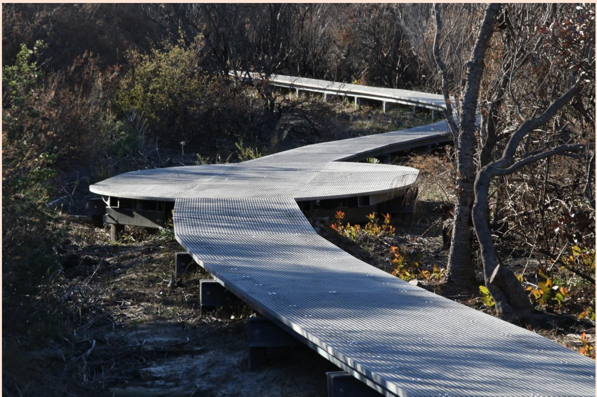
Note the clean lines along the edges of the track to protect it from the burn
