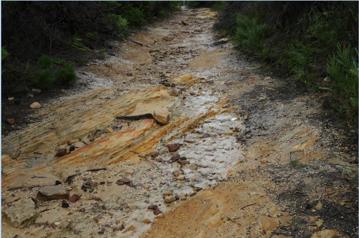
Track without good drainage
